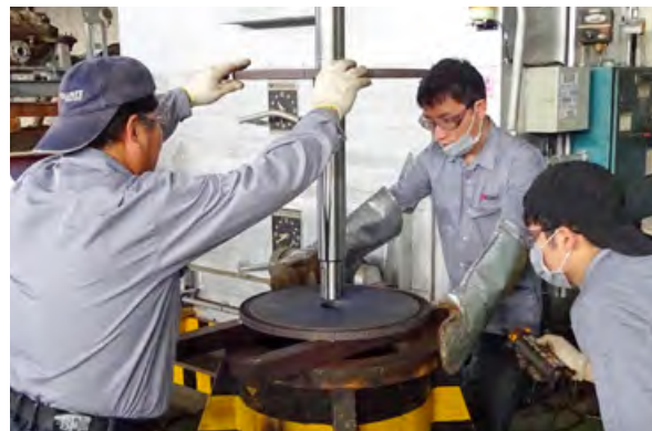
New shaft installation.
