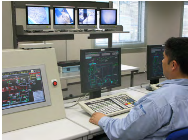
Monitoring and data analysis during testing.
