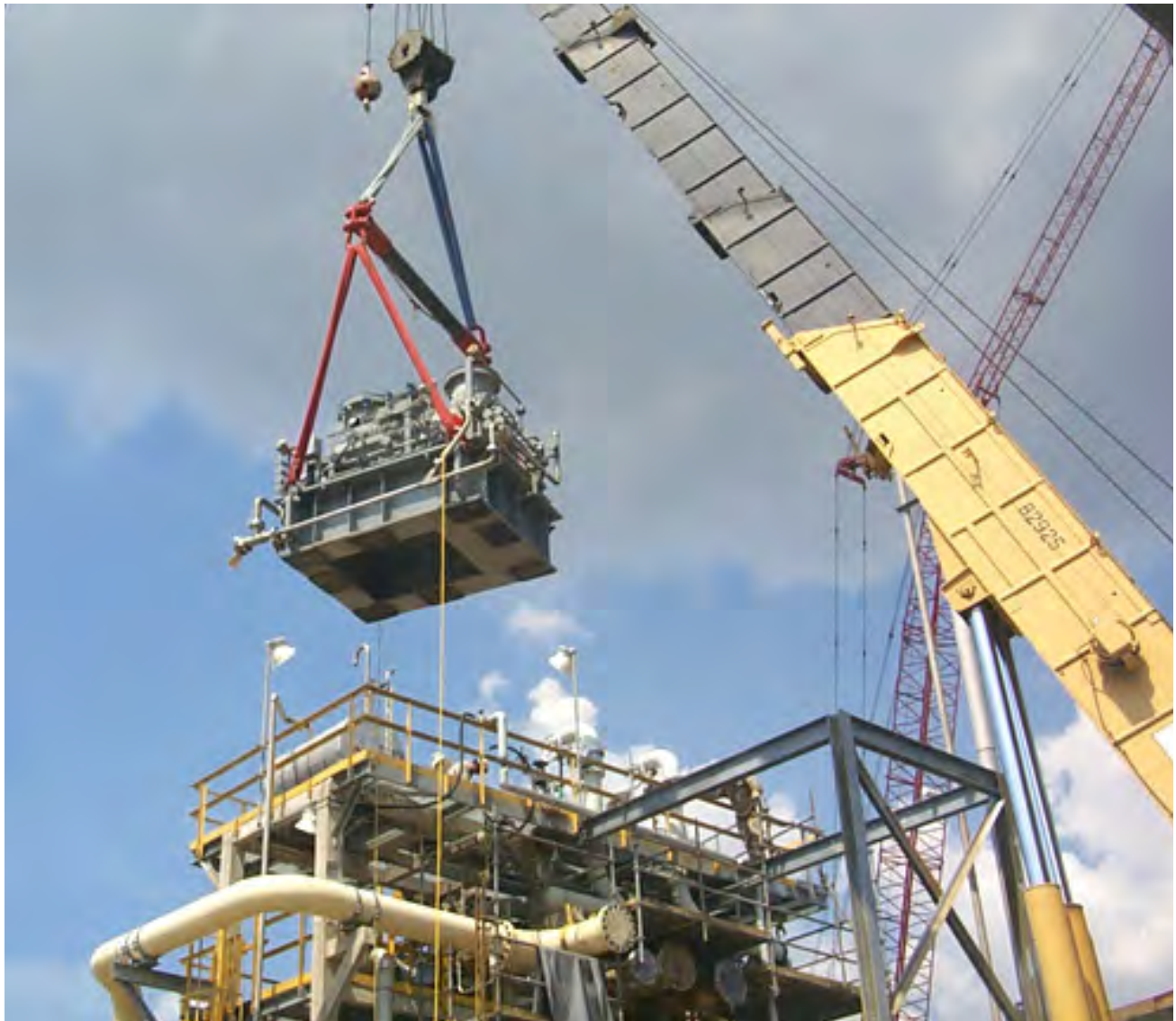
Installation, commissioning, and start-up services.
