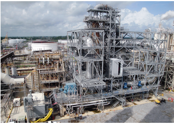
Figure 3. FCC regenerator in a US refinery. An Elliott TH-140 expander gear generator train are in the center on the first deck.
