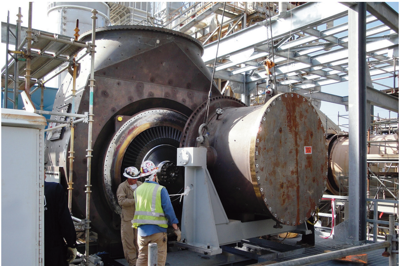
Figure 5. Removing the inlet casing to access the expander rotor.
