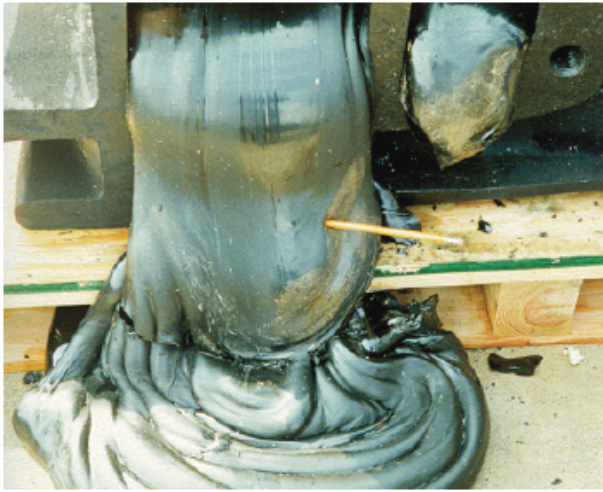
Figure 1. Foulant build up from a compressor.
