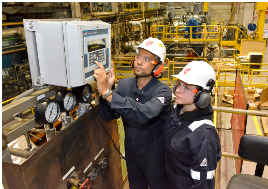
Cover Photo: Two Elliott employees program a Woodward 505 Governor Control which provides electronic speed and trip control for a turbine.
