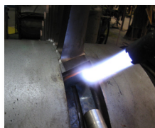
Blades being removed from rotor shaft.
